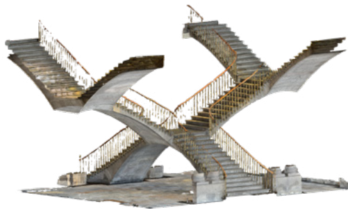
FIGURE 6. Staircase, MNH. 3D model elaborated by digital photogrammetry (Survey and model elaboration: Fabián Bernal Orozco Barrera, January 16, 2023; courtesy: Museo Nacional de Historia, CNMH).
