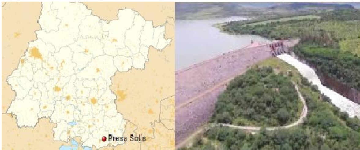
Figure 1. Location of the Solís dam (Conagua, 2016).
